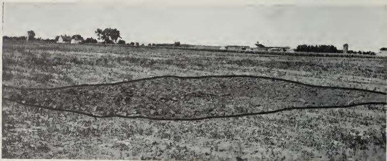
FIG. 37.—Pit holes near Streator caused by room-and-pillar mining filled with mine rock and surfaced with soil. The dark lines border the area of filling.
